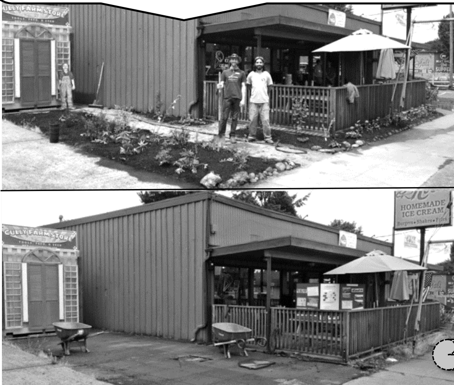
Bottom picture: shop with pavement driveway (where wheelbarrows are); Top picture: pavement removed and soil and plants added! (Image from Depave).
