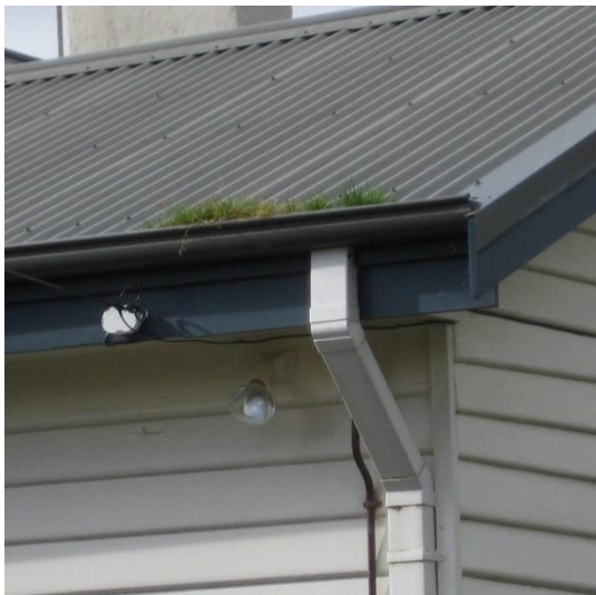
Gutter / Downspout
