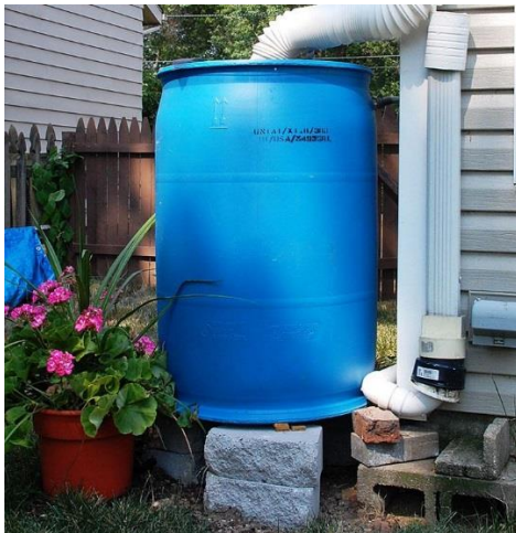
Rain Barrel or Cistern
